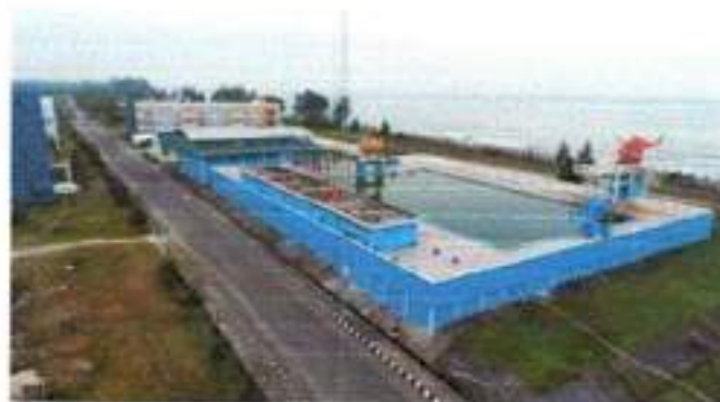
Gambar 4. 17 Gedung Water Pit
