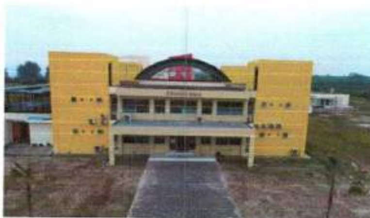
Gambar 4. 23 Gedung Dinning Hall
