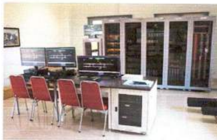
Gambar 4. 56 Central Base Interlocking
