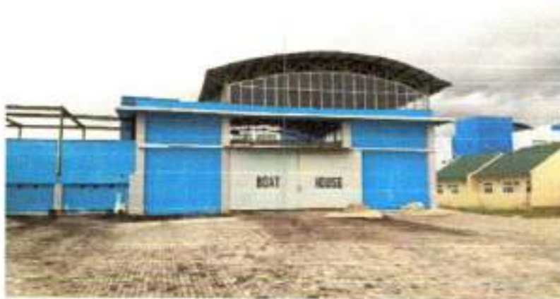
Gambar 4. 21 Gedung Boat House
