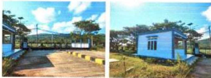
Gambar 4. 27 Main Entrance Tahap I
